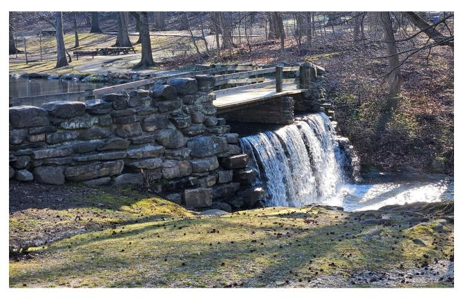
Walk along the entire crest of the dam, looking for deficiencies including but not limited to, erosion, settlement, and movement or misalignment. Make note of the vegetative condition and look for signs of seepage.
