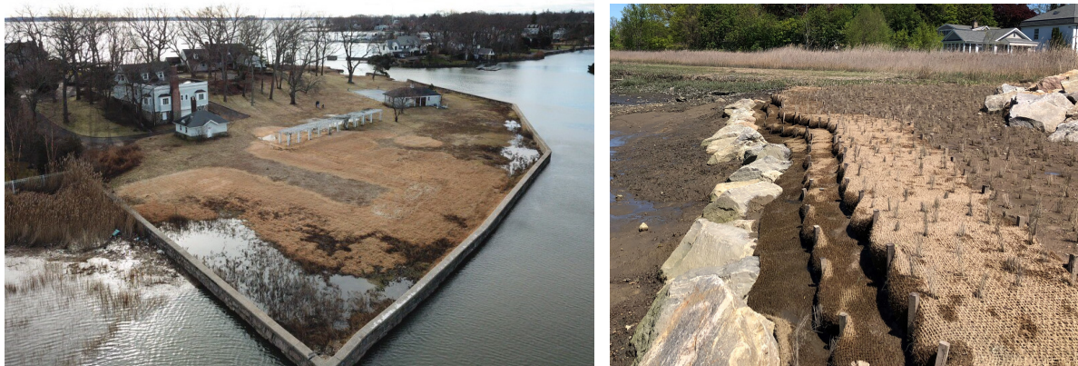
Figure 17. Vertical Seawall in the Process of Being Replaced with a Nature-Based Shoreline (left vertical seawall before construction, right the terraced design and native plantings following construction.) Photos courtesy of Bryan Martin and Angela Schimizzi
