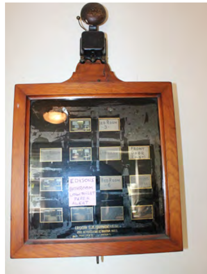
Figure II-316. Original servant's call annunciator box in Servant's Hall (118). (HA, 2015)
