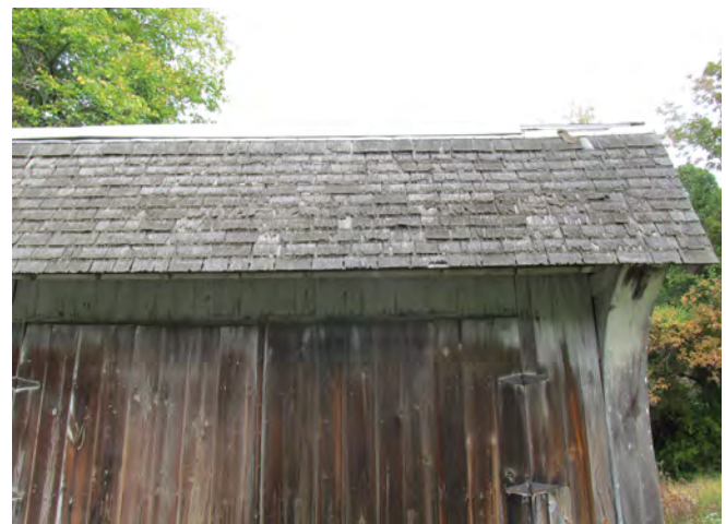
Figure IV-177. Worn and displaced roof shingles on south slope. (HA, 2015)
