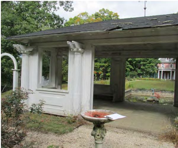
Figure II-110. Damaged garden house roof edge and missing gate. Looking north from rose garden. (HA, 2015)
