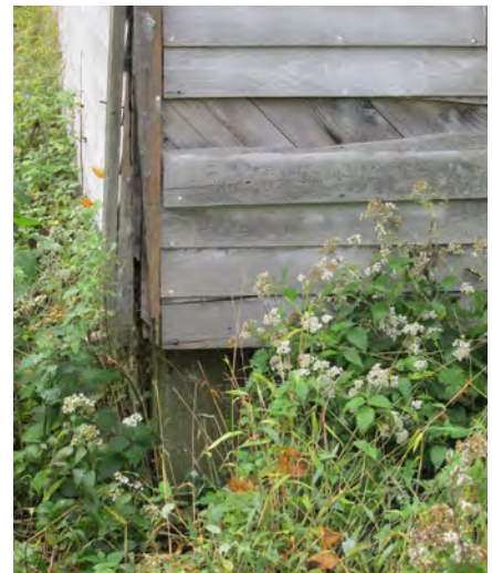
Figure IV-171. Damaged clapboard siding. (HA, 2015)
