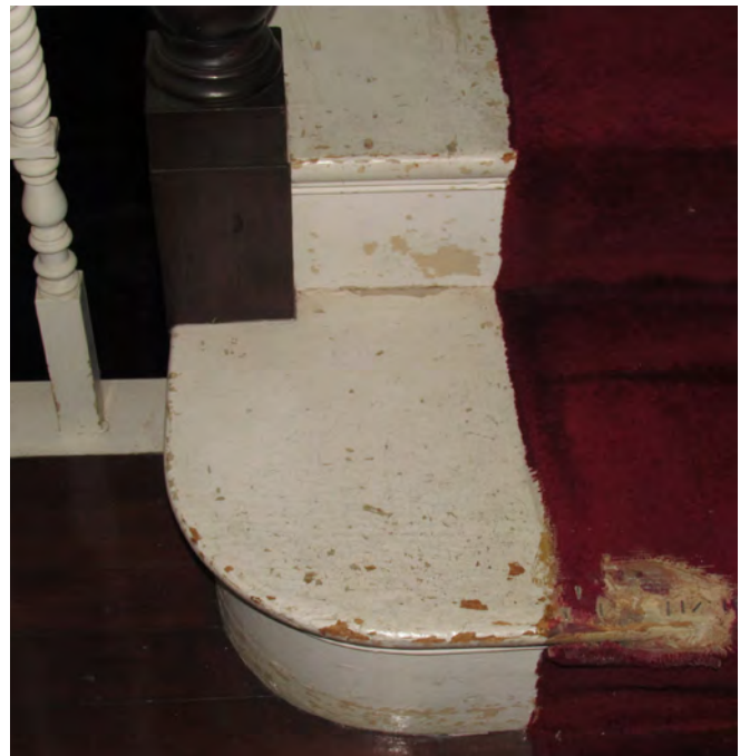
Figure II-240. Scratches and nicks at main stair painted treads and risers. (HA, 2015)
