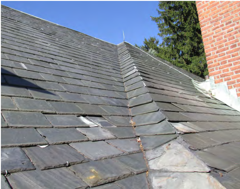
Figure II-148. Slate roof showing eroded and missing tiles. (HA, 2015)
