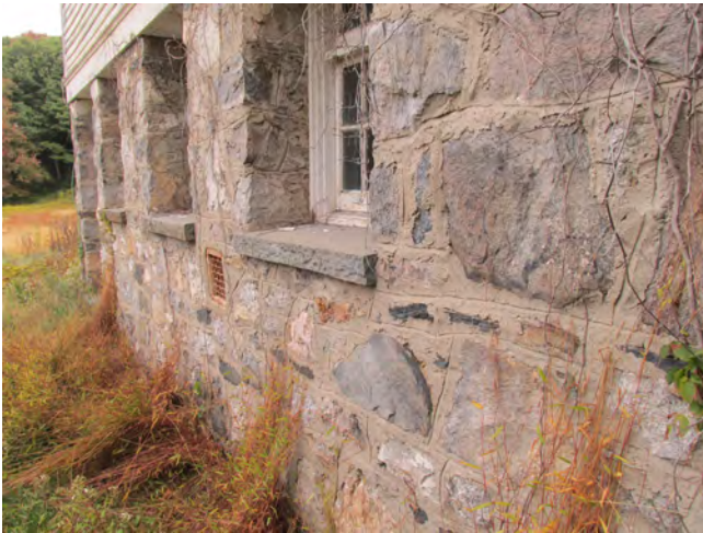
Figure IV-95. Fieldstone foundation wall. (HA, 2015)
