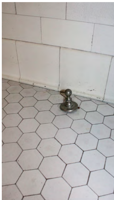
Figure II-237. Ceramic tile base. (HA, 2015)
