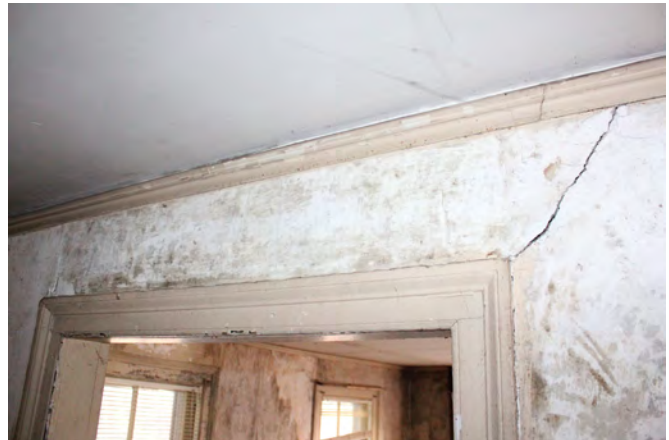
Figure IV-48. Plaster crack in plaster above salon/living room mantle piece in 19th century section of the house. (HA, 2015)
