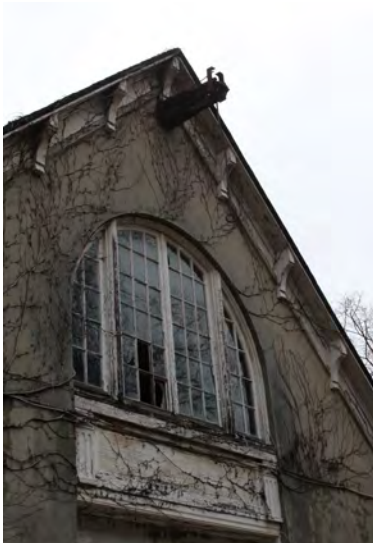
Figure III-45. Multiple-lite casement windows and flanking fixed windows at south elevation. (HA, 2015)
