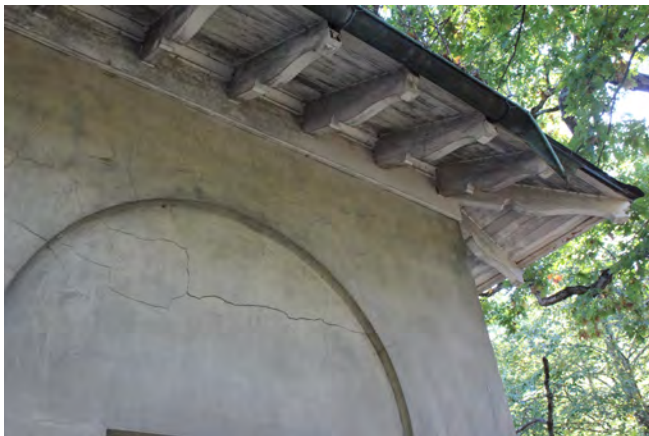
Figure III-31. Cracks in stucco. (HA, 2015)
