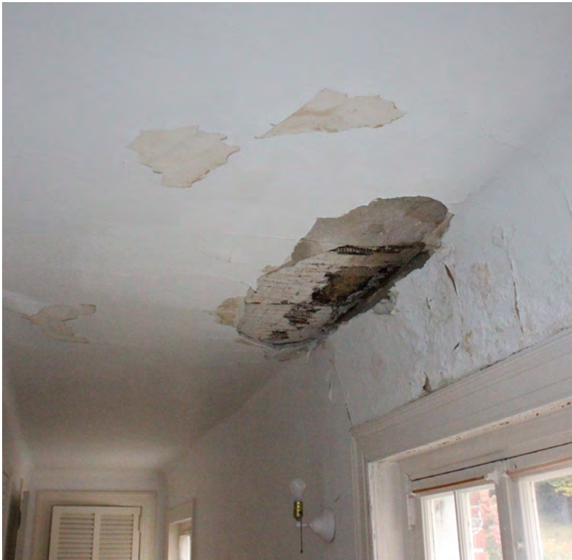
Figure II-232. Plaster and paint failure due to water infiltration in Servant's Corridor (224). (HA, 2015)
