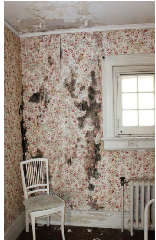
Figure II-233. Mold growth, water staining and peeling paint and wallpaper in Servant's Bedroom D (222). (HA, 2015)
