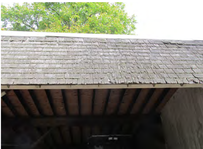
Figure IV-176. Worn and displaced roof shingles on south slope. (HA, 2015)
