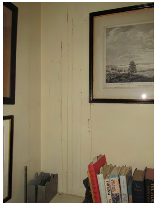
Figure II-231. Staining/drip marks on Bedroom 1 (216) wall. (HA, 2015)
