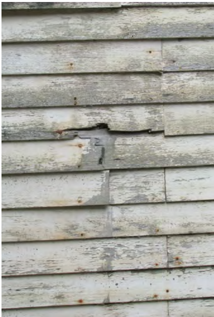
Figure IV-132. Worn paint finish and damaged clapboard. (HA, 2015)
