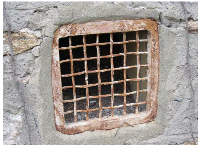
Figure IV-104. Corroded metal vent in fieldstone walls. (HA, 2015)
