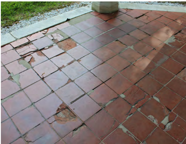
Figure II-128. Deteriorated clay tile at porch. (HA, 2015)
