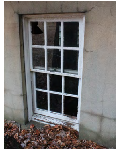
Figure III-119. 6/6 double-hung window. (HA, 2015)
