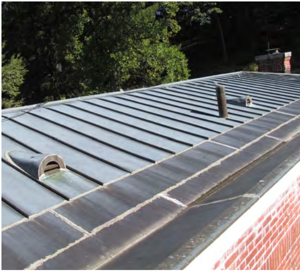
Figure II-152. Standing seam copper roof with flat seam gutter liner over the servant's wing. (HA, 2015)
