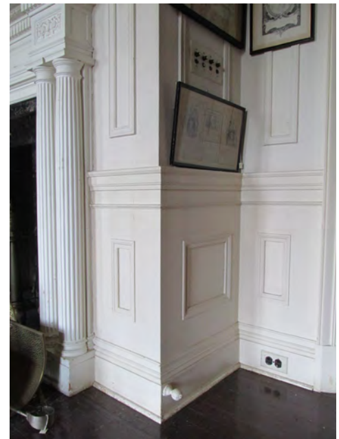
Figure II-218. Panelized walls in the Dining Room (108). (HA, 2015)
