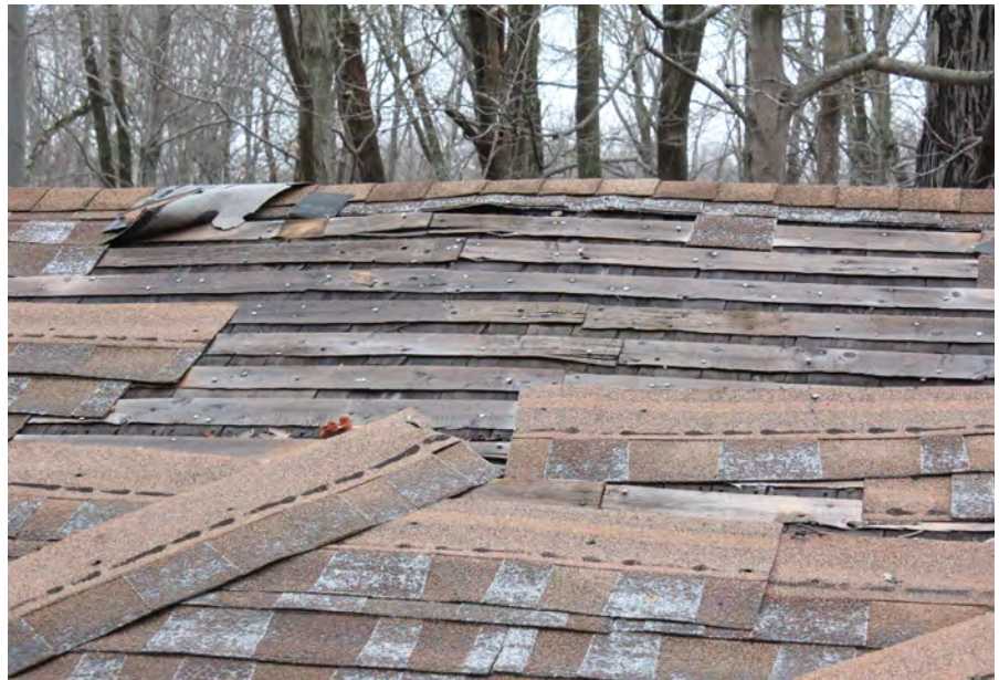
Figure III-135. Missing and loose asphalt shingles. (HA, 2015)
