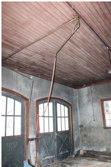
Figure III-127. Ceiling mounted hose arm. (HA, 2015)
