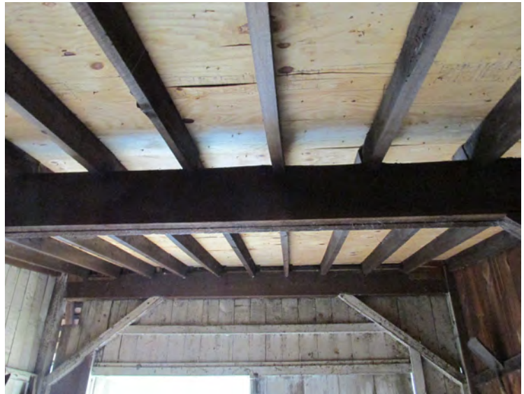
Figure IV-181. Exposed wood roof framing and plywood sheathing. (HA, 2015)
