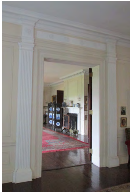
Figure II-254. Pilasters framing doorways to Dining and Living Rooms. (HA, 2015)
