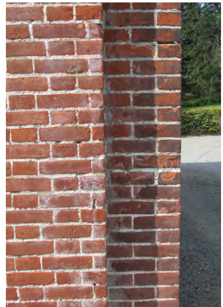
Figure II-132. Eroded brick mortar joints and soft brick. (HA, 2015)
