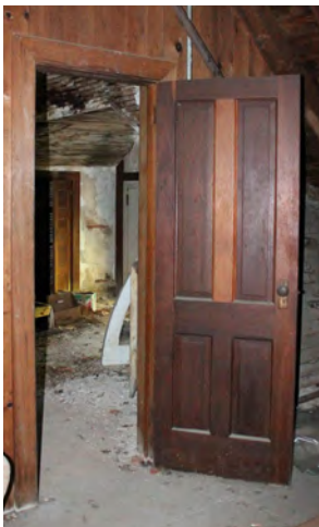
Figure III-74. Four-paneled door. (HA, 2015)
