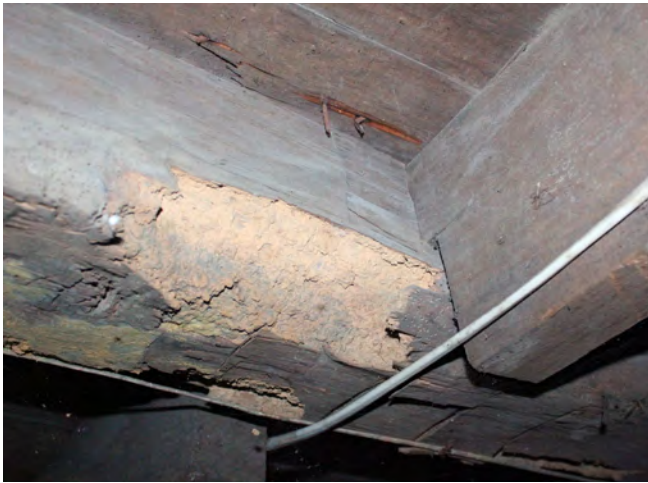
Figure IV-79. Heavy timber floor beams in 19th century section of the house. Termite damage has caused significant damage to some of the members. (HA, 2015)
