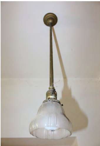
Figure II-304. Light fixture type L13; Bronze or brass single light hanging pendant with glass shade. (HA, 2015s)
