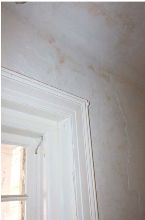
Figure II-226. Chipped paint and water staining at exterior wall in Servant's Corridor (115). (HA, 2015)
