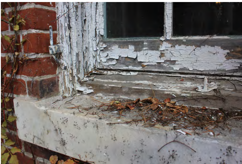
Figure II-173. Paint failure at windows. (HA, 2015)
