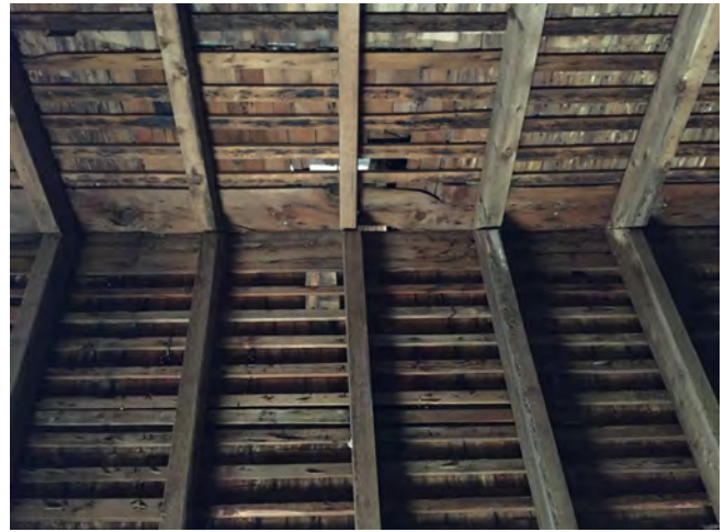
Figure IV-152. Exposed roof framing and sheathing in hayloft. (HA, 2015)
