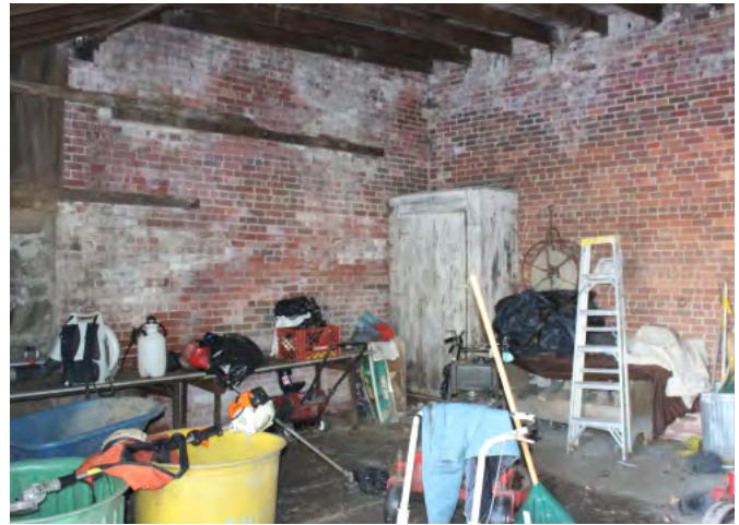
Figure II-122. Interior of garage/shed showing extensive efflorescence on brick walls. (HA, 2015)
