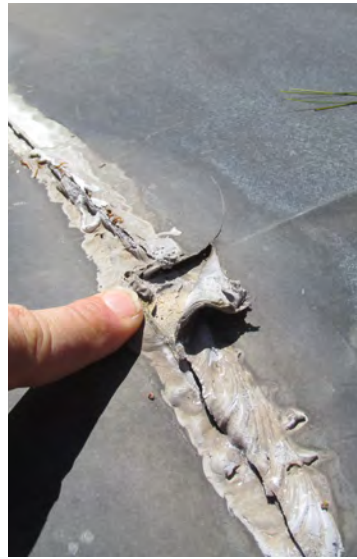
Figure II-153. Failed solder joint at flat seam gutter on servant's wing. (HA, 2015)
