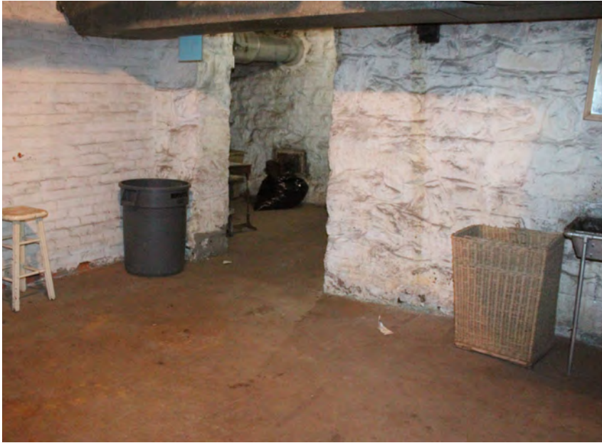
Figure II-213. Brick (left) and stone rubble (right) walls in the basement. (HA, 2015)
