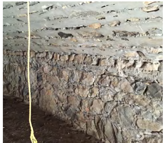
Figure IV-217. Close-up photo of fieldstone walls and barrel ceiling. (HA, 2015)
