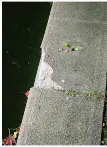
Figure II-114. Damaged concrete swimming pool coping unit. (HA, 2015)
