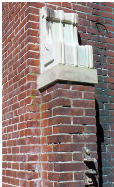
Figure II-131. Eroded brick mortar joints. (HA, 2015)
