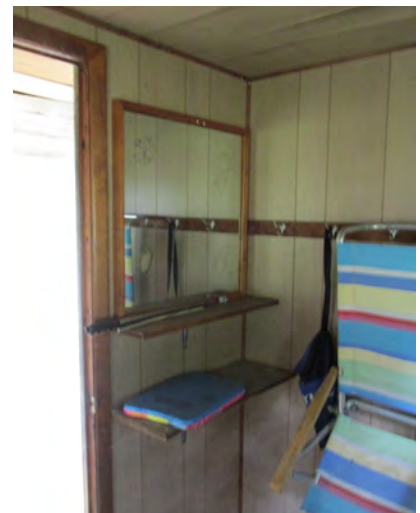
Figure II-120. Changing room mirror and shelf. Note paneling on ceiling is loose/displaced. (HA, 2015)
