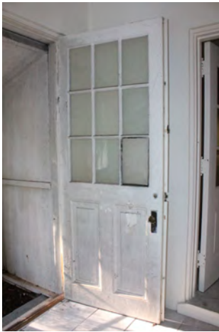
Figure III-78. Nine lite, two-paneled door. (HA, 2015)
