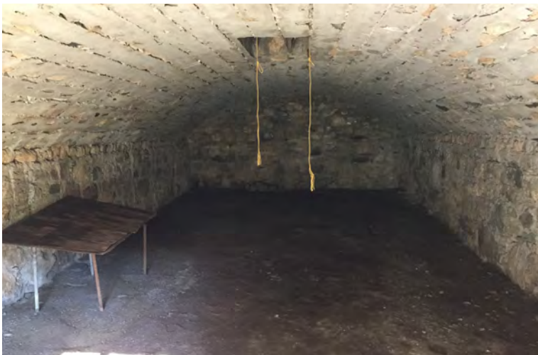
Figure IV-216. Fieldstone walls and barrel ceiling. (HA, 2015)
