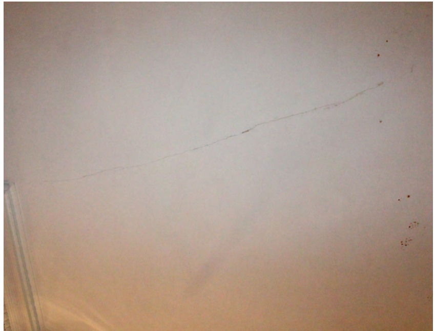
Figure II-222. Ceiling crack in the Living Room (106) ceiling (HA, 2015)
