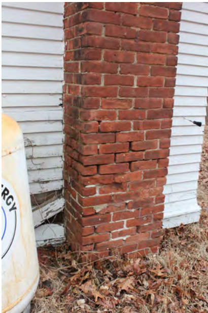
Figure III-134. Siding damage and loss of masonry mortar. (HA, 2015)
