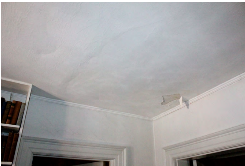
Figure II-234. Crazed and peeling paint at third floor Hall (301) ceiling. (HA, 2015)
