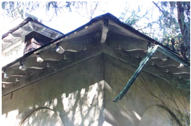
Figure III-54. Missing and damaged copper gutters. (HA, 2015)
