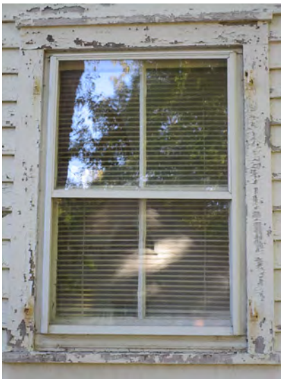
Figure IV-33. 2/2 double-hung window in 19th century section of the house with aluminum storm window. (HA, 2015)
