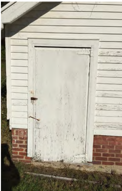
Figure IV-186. Painted plywood has been installed over the exterior of the stile and rail door. (HA, 2015)
