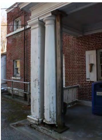
Figure II-318. Additional wood posts used to support north servant's porch. (HA, 2015)
