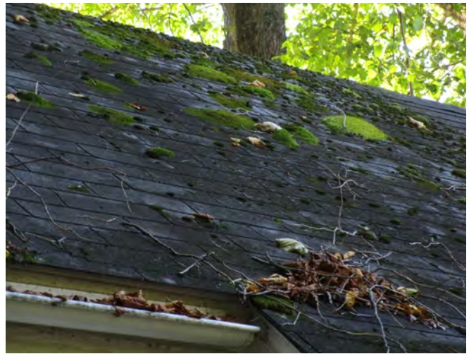
Figure IV-163. Worn shingles and biological growth and debris on roof. (HA, 2015)
