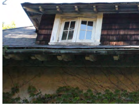
Figure III-46. Four-lite casement at dormers. (HA, 2015)
