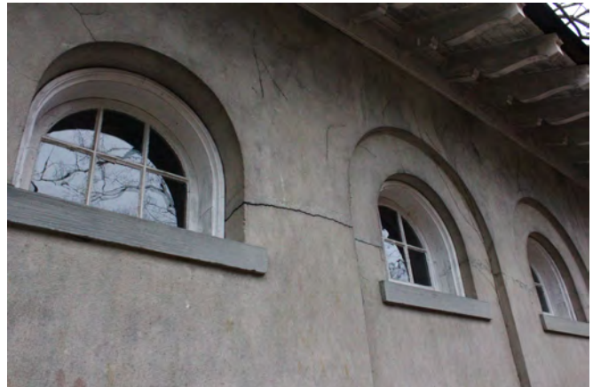
Figure III-32. Cracks in stucco. (HA, 2015)
