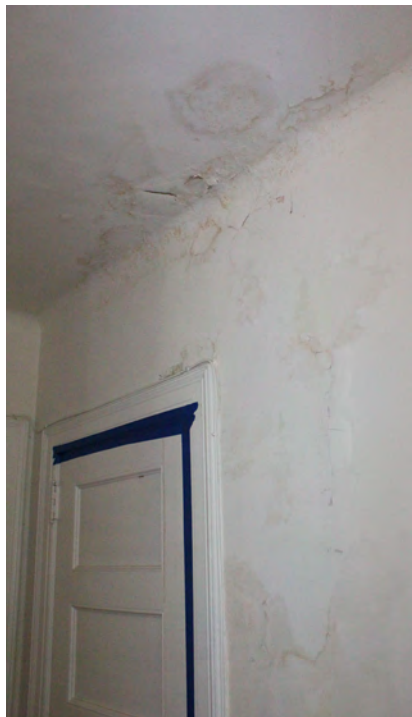
Figure II-227. Delaminated plaster and water staining in Laundry Room (119). (HA, 2015)
