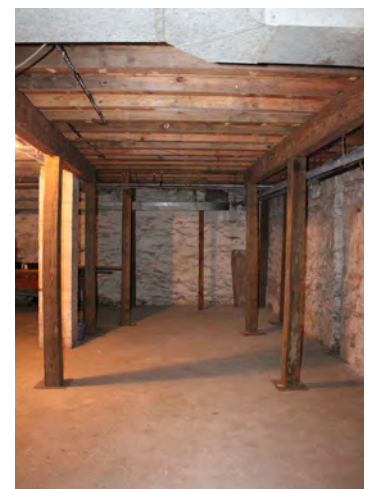
Figure II-320. Additional wood posts installed in the basement to reinforce dining room floor. (HA, 2015)
