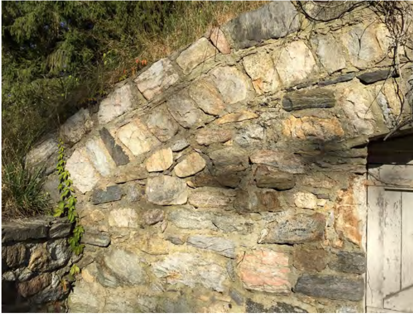
Figure IV-210. Fieldstone root cellar wall. (HA, 2015)
