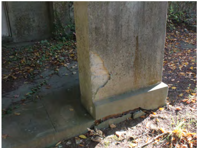
Figure III-28. De-laminated concrete at porch column base. (HA, 2015)
