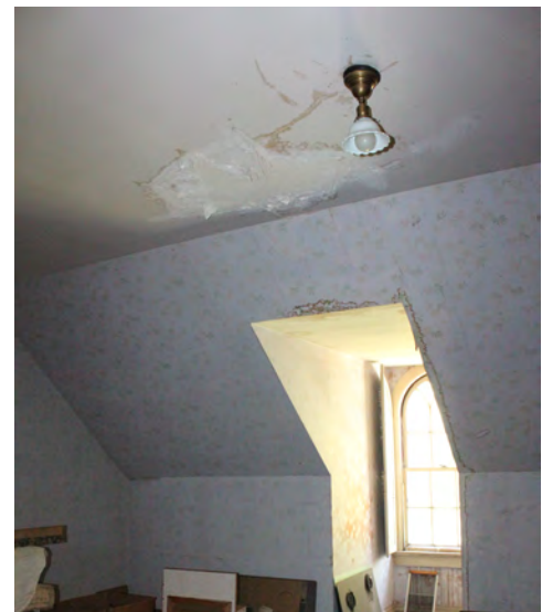
Figure II-235. Water staining and peeling paint in Bedroom 9 (307). (HA, 2015)
