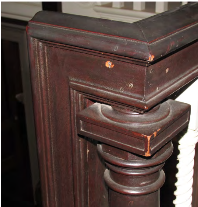
Figure II-239. Holes and scratches at main stair handrail. (HA, 2015)
