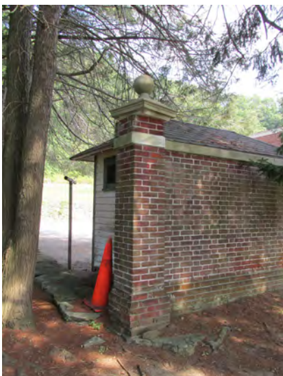
Figure II-106. Displaced marble finial cap at brick masonry end post (Image from Harboe Architects).
