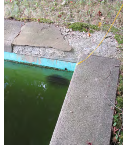
Figure II-115. Damaged concrete swimming pool coping unit. (HA, 2015)
