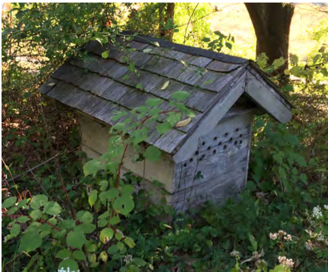
Figure IV-214. Earth roof and wood ventilator with wood roof shingles at lower root cellar. (HA, 2015)
