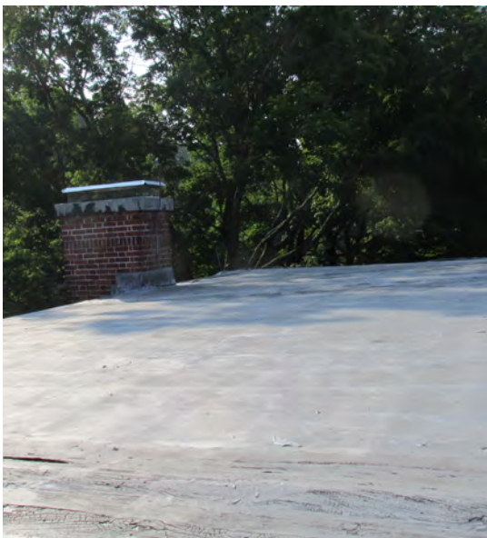
Figure II-150. Asphaltic roofing at flat roof over house, looking southeast. (HA, 2015)
