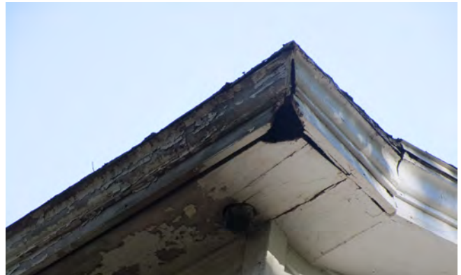
Figure IV-40. Loose and damaged soffit boards. (HA, 2015)
