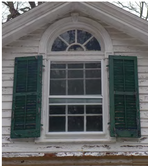
Figure IV-34. 6/6 double-hung window with fan lite above and aluminum storm window. (HA, 2015)
