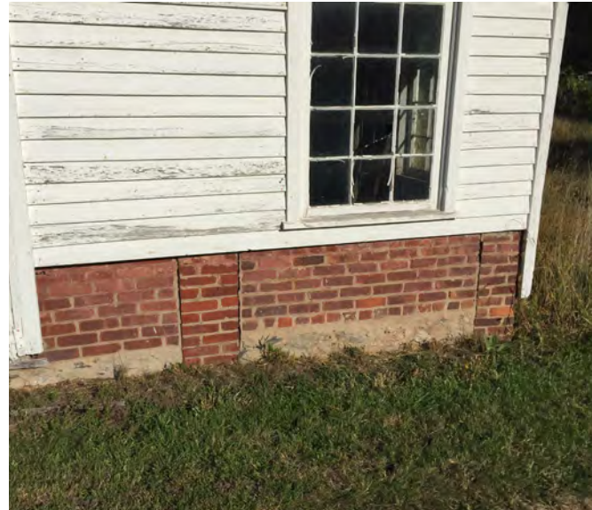
Figure IV-185. Brick piers with later brick infill at foundation. (HA, 2015)
