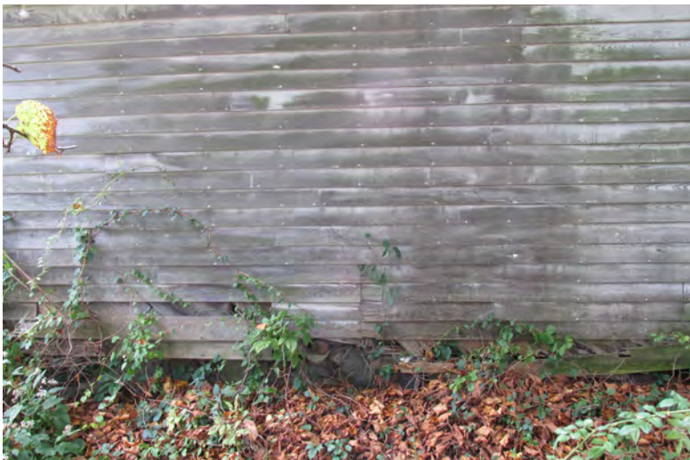
Figure IV-170. Worn paint finishes and damaged clapboard siding. (HA, 2015)
