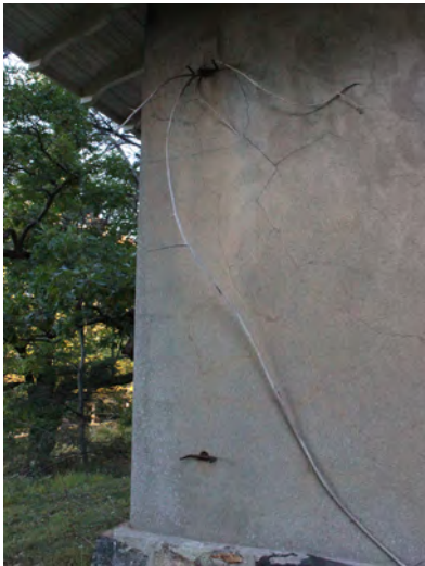
Figure III-117. Cracks in stucco. (HA, 2015)
