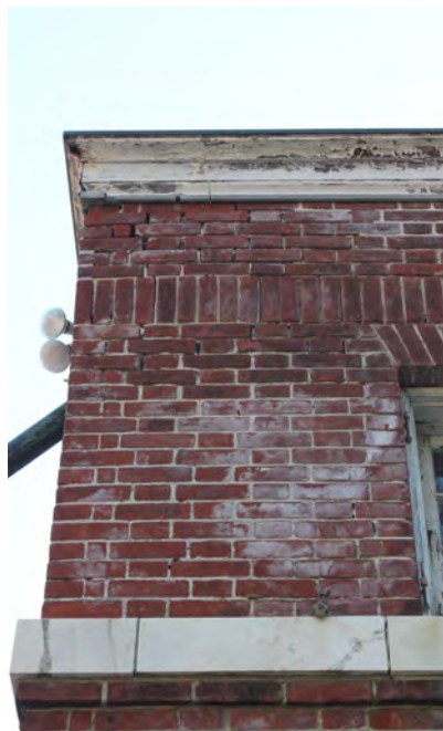
Figure II-134. Efflorescence on north elevation of servant's wing (HA, 2015)
