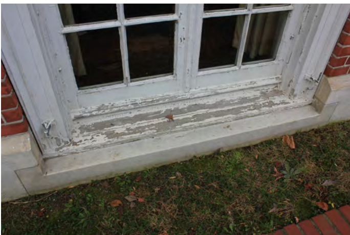
Figure II-164. Severely worn wood sill at French doors. (HA, 2015)
