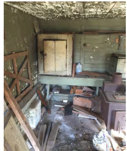
Figure IV-192. Peeling paint at plaster walls and wood ceiling. (HA, 2015)
