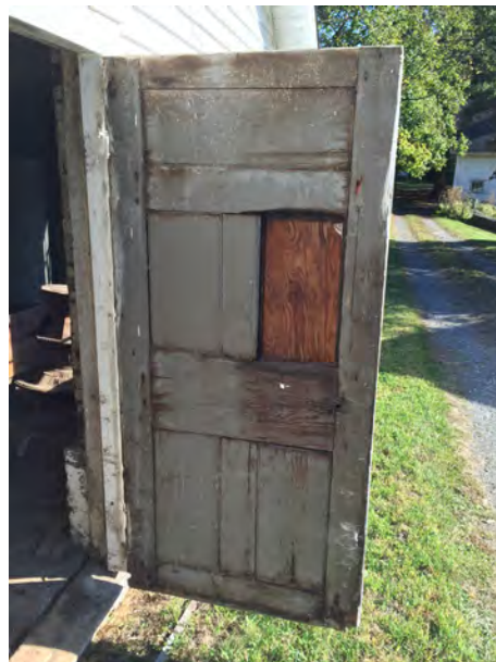
Figure IV-187. Interior face of the stile and rail door. (HA, 2015)
