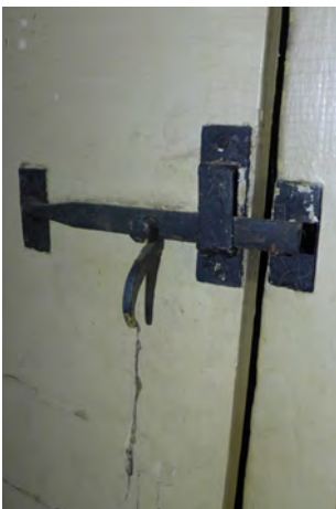
Figure IV-65. Iron Suffolk latch in 19th century section of house. (HA, 2015)
