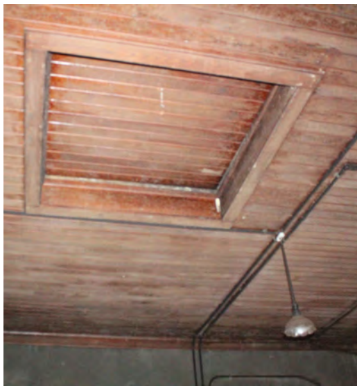
Figure III-124. Roof hatch and pendant light. (HA, 2015)
