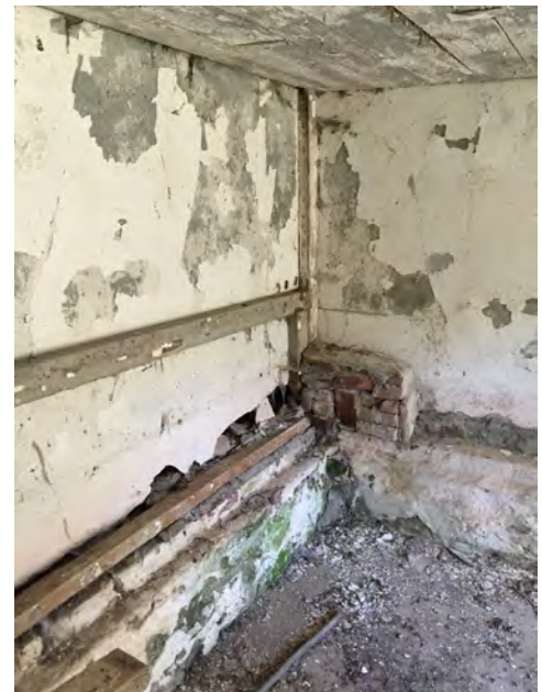
Figure IV-194. Delaminated and spalled plaster walls.. (HA, 2015)
