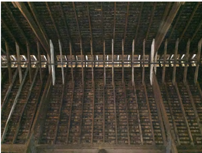
Figure IV-113. Exposed roof structure on upper level. The walls are likewise not clad but rather reveal the structural framing and backside of wood sheathing. (HA, 2015)
