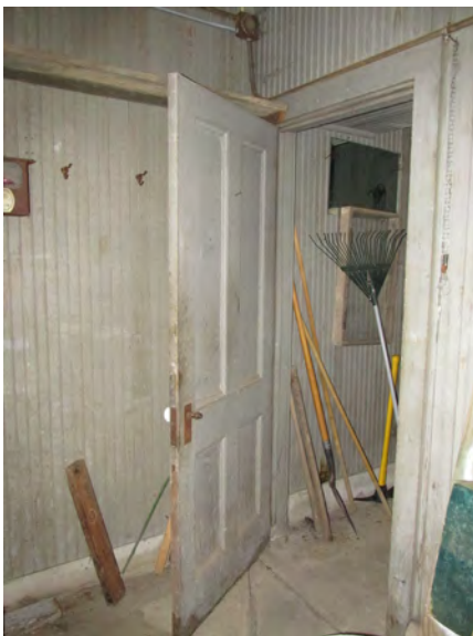
Figure IV-153. Painted four-panel wood door. (HA, 2015)
