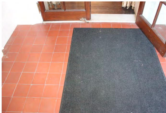
Figure II-200. Quarry tiles in Vestibule (101). (HA, 2015)
