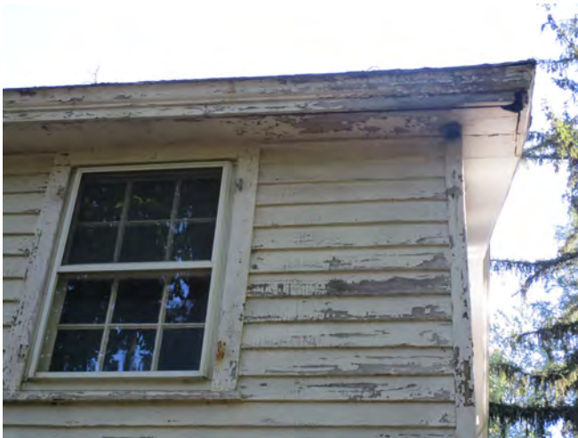
Figure IV-28. Paint failure on clapboard siding. (HA, 2015)
