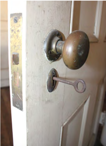
Figure IV-61. Lockset with bronze knob, rosette, and skeleton key escutcheon plate. Lockset likely dates from early 20th century. (HA, 2015)
