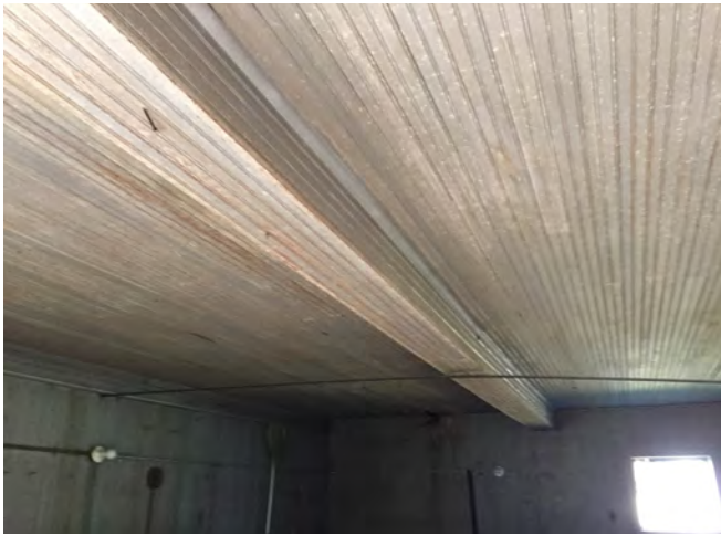
Figure IV-151. Painted tongue-and-groove ceiling boards in garage and horse stall area. (HA, 2015)
