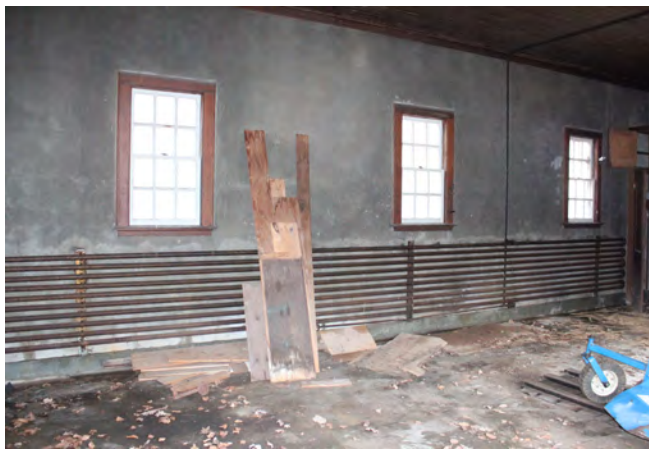
Figure III-122. Hot water pipes along west wall. (HA, 2015)
