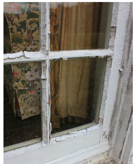
Figure II-174. Failing glazing putty. (HA, 2015)
