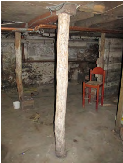
Figure IV-81. Wood post in basement of 19th century house. The wood post essentially consists of a tree branch that was minimally hewed. (HA, 2015)
