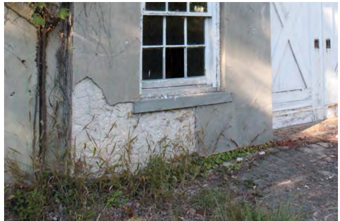
Figure III-34. Missing stucco near carriage room doors. (HA, 2015)
