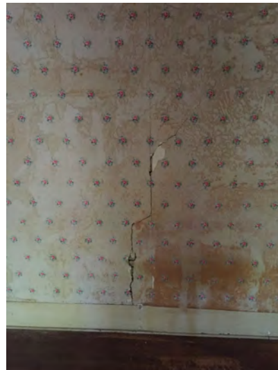
Figure IV-50. Cracks in plaster wall. (HA, 2015)
