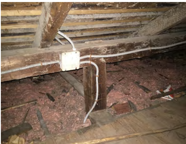
Figure IV-83. Heavy timber knee wall in western half of 19th century attic. The knee wall may represent the oldest portion of the house and was made popular during the advent of the Greek Revival style in the mid 19th century. (HA, 2015)
