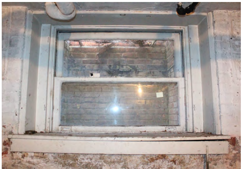
Figure II-170. 1/1 double-hung window in basement. (HA, 2015)
