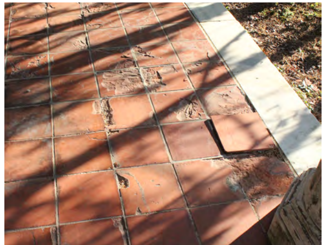
Figure II-129. Deteriorated clay tile at porch. (HA, 2015)
