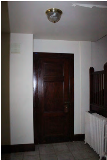
Figure III-101. Surface mounted ceiling light fixture. (HA, 2015)
