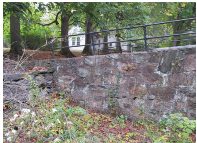
Figure IV-98. Fieldstone ramp walls and metal railings with connection fittings. (HA, 2015)
