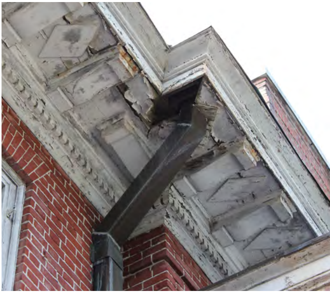
Figure II-138. Rotted wood soffit at downspout. (HA, 2015)
