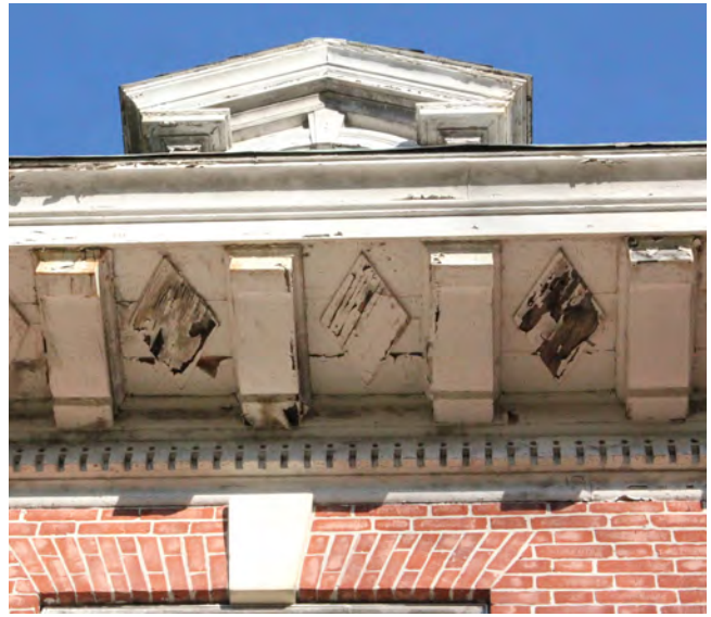
Figure II-139. Paint failure and rotted wood soffit elements. (HA, 2015)
