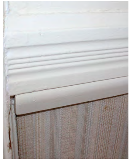
Figure II-250. Chair rail used in the Servant's Hall (118). (HA, 2015)
