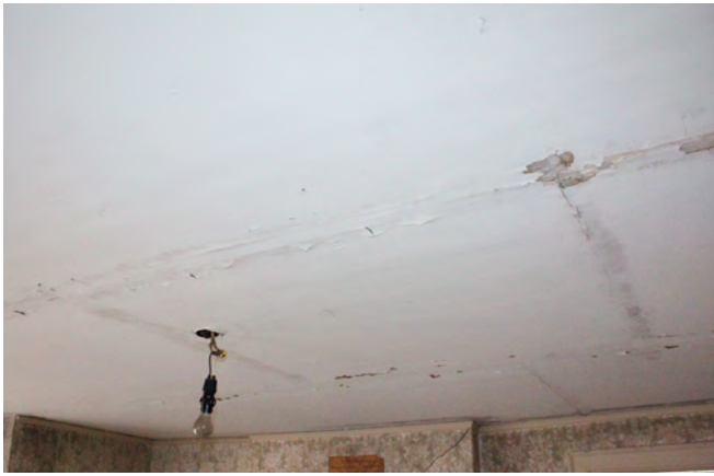
Figure IV-52. Patches in ceiling plaster and peeling paint in 19th century section of the house. (HA, 2015)
