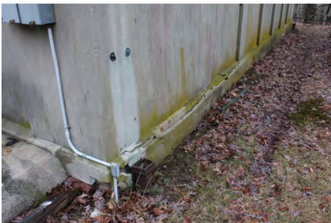
Figure III-33. De-laminated stucco at base. (HA, 2015)
