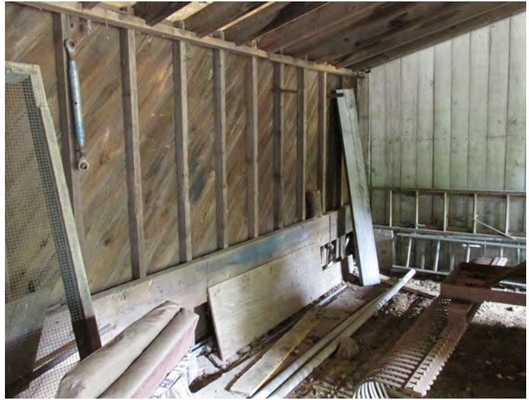
Figure IV-179. Exposed wood framing and diagonal wood sheathing of perimeter walls. (HA, 2015)
