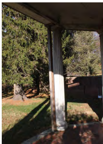
Figure II-319. Additional wood posts used to support north porch. (HA, 2015)
