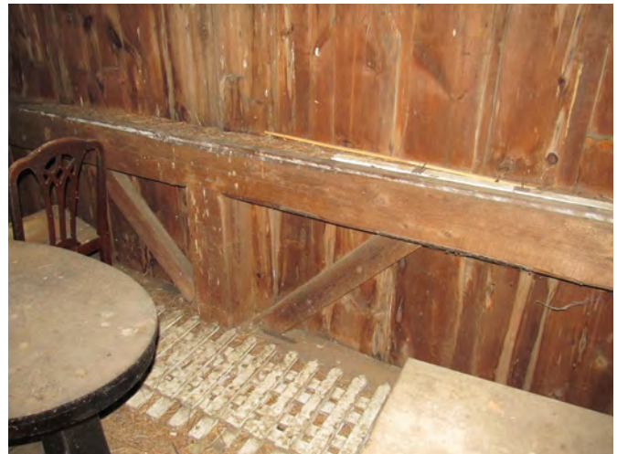
Figure IV-150. Exposed heavy timber framing and wood sheathing in hayloft. (HA, 2015)
