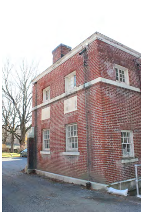
Figure II-156. Missing copper downspouts at east elevation servant's wing. (HA, 2015)
