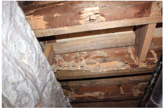
Figure II-322. Termite damaged floor joists under the dining room. (HA, 2015)
