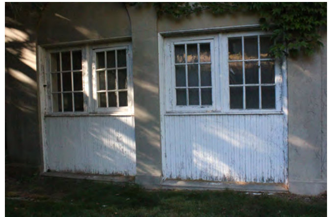
Figure III-36. Wood partition in-fill walls at enclosed porch. (HA, 2015)
