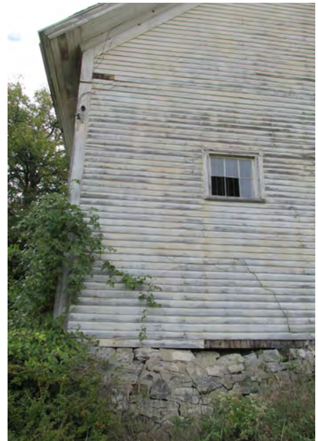
Figure IV-134. Displaced foundation stones. (HA, 2015)
