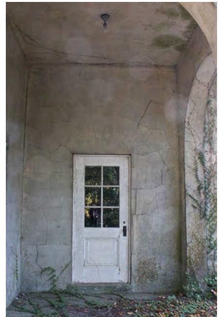
Figure III-57. Missing pendant light fixture at east porch. (HA, 2015)
