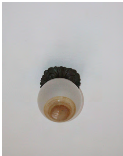
Figure II-293. Light fixture type L2; Ceiling fixture with painted metal decorative base and glass obscure glass shade. (HA, 2015)
