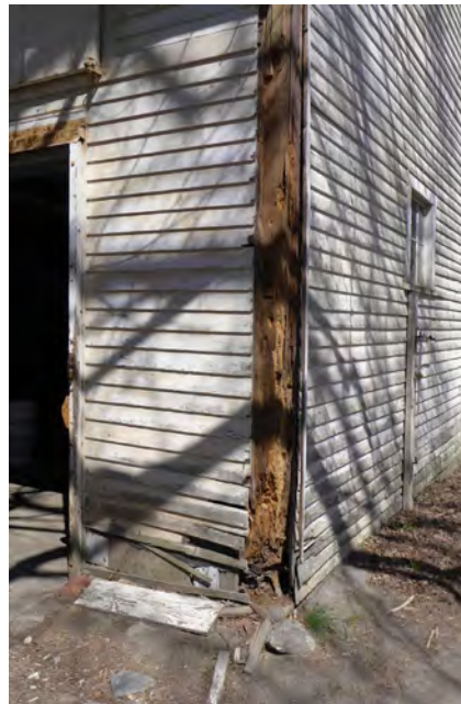
Figure IV-133. Missing corner board and clapboard siding at southeast corner. The corner post also has significant termite damage. (HA, 2015)
