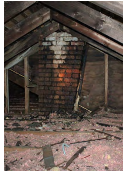
Figure IV-43. Chimney at eastern portion of the 19th century house section. Chimney was capped off below the roof line. (HA, 2015)
