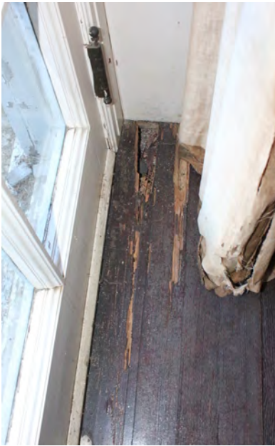
Figure II-206. Termite damage in Dining Room (108). (HA, 2015)
