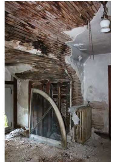
Figure III-66. Plaster damage in groom's bedroom. (HA, 2015)
