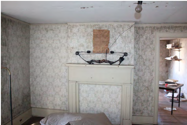
Figure IV-47. Plaster crack in plaster above salon/living room mantle piece in 19th century section of the house. (HA, 2015)
