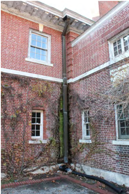
Figure II-155. Copper downspout at intersection of house and servant's wing. Note, downspout not connected to a drainage pipe. (HA, 2015)
