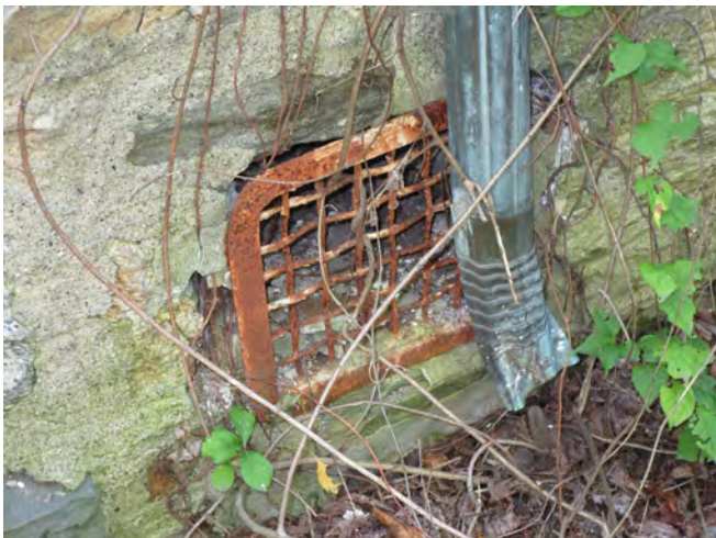
Figure IV-103. Corroded metal vent in fieldstone walls. (HA, 2015)
