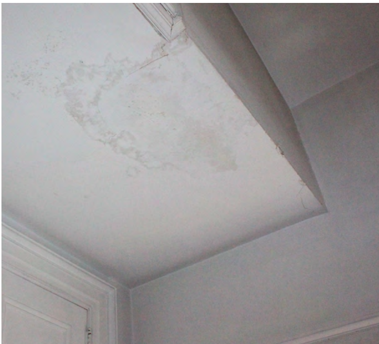
Figure II-230. Water staining at third floor Stair (204) ceiling. (HA, 2015)
