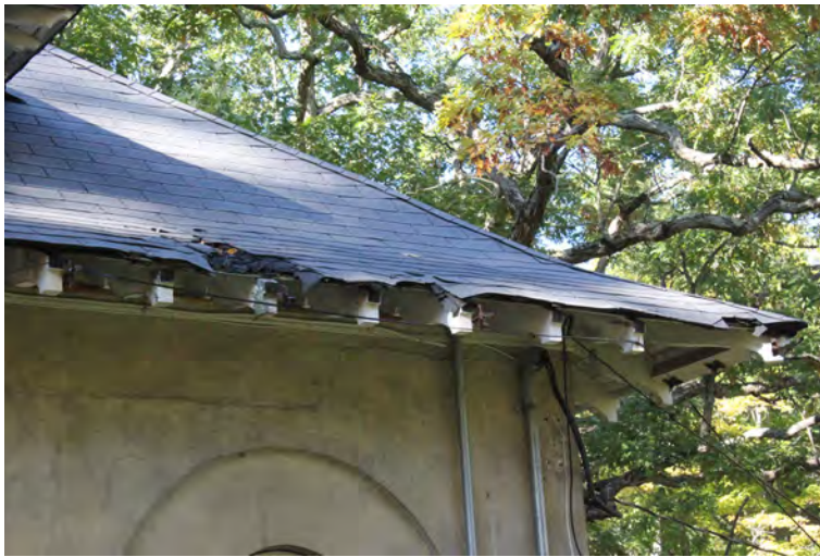
Figure III-51. Impact damage to asphalt shingles. (HA, 2015)
