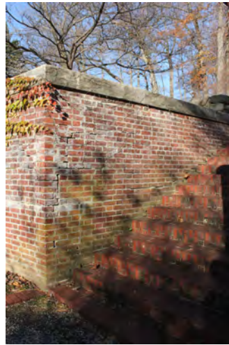
Figure II-102. Displaced brick, eroded mortar joints, and efflorescence at retaining wall. (HA, 2015)
