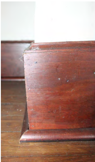
Figure III-82. Typical base molding. (HA, 2015)
