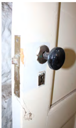
Figure II-278. Lockset with black porcelain knob, used in basement. (HA, 2015).
