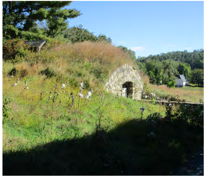
Figure IV-213. Earth roof at upper root cellar. (HA, 2015)
