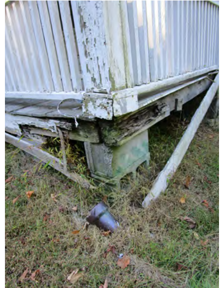
Figure IV-38. Close-up of rotted and missing wood at southeast corner of porch as well as added CMU corner support. (HA, 2015)
