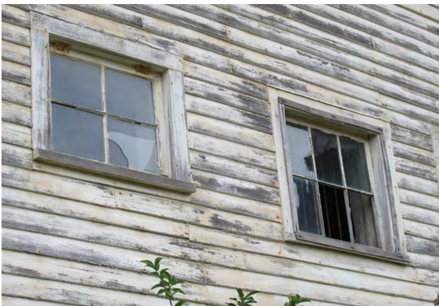
Figure IV-140. Four and six-light painted wood windows. (HA, 2015)
