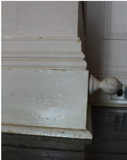
Figure II-245. Base molding used in Dining (108) and Living (106) Rooms. (HA, 2015)
