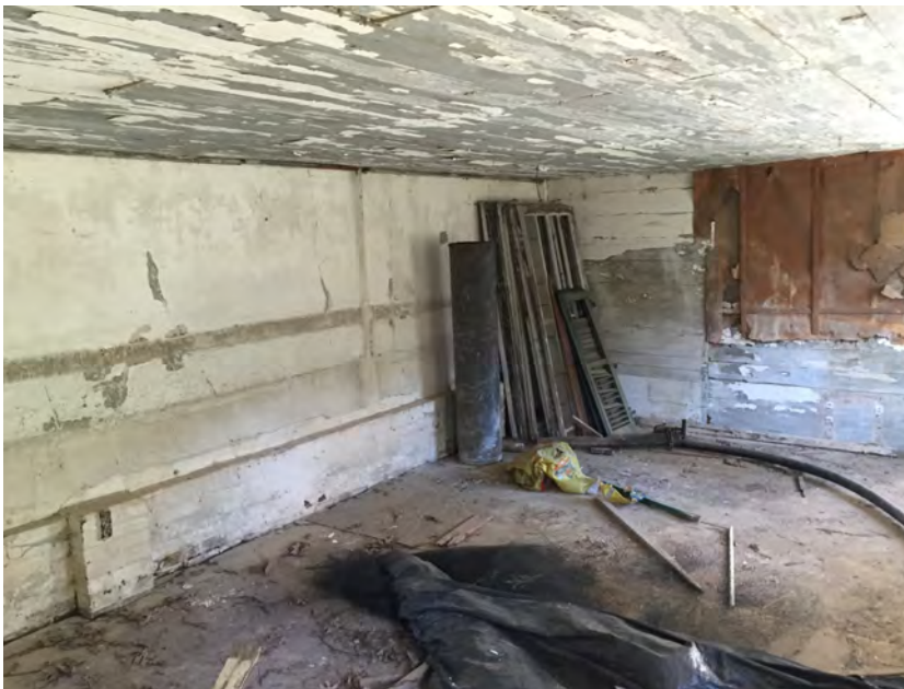
Figure IV-193. Peeling paint at walls and ceiling. (HA, 2015)
