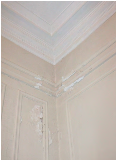
Figure II-221. Peeling paint and plaster damage in Hall (107). (HA, 2015)
