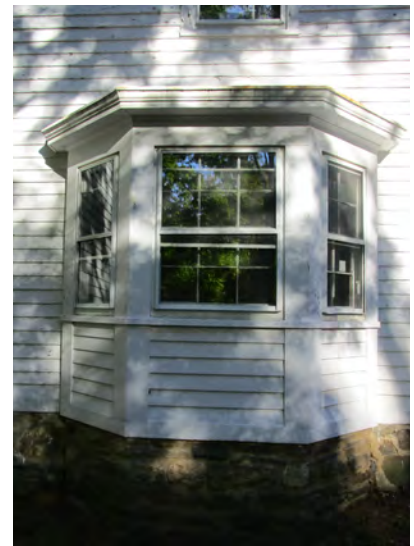
Figure IV-35. 6/6 and 4/4 double-hung windows in bay addition of 19th century section of the house. (HA, 2015)
