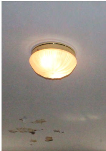
Figure II-305. Light fixture type L14; Brass ceiling mounted fixture with glass schoolhouse dome. (HA, 2015)
