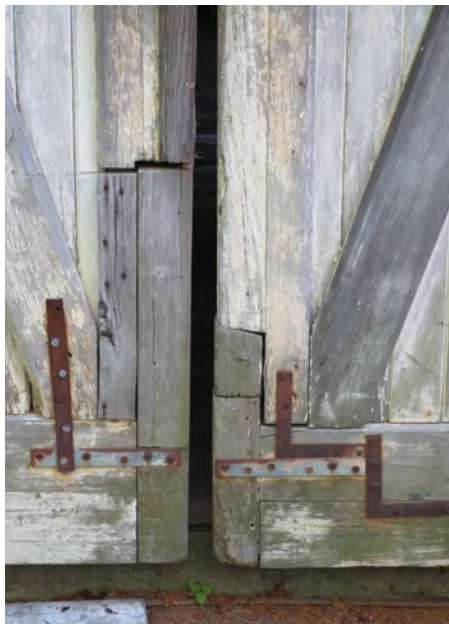
Figure IV-99. Metal strap reinforcing at main barn doors. (HA, 2015)
