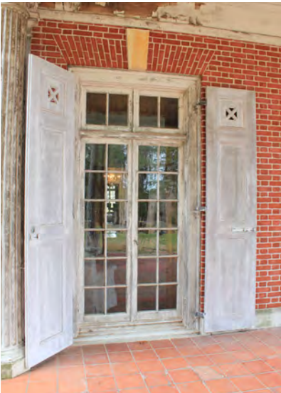
Figure II-161. French doors and transom at north porch. (HA, 2015)
