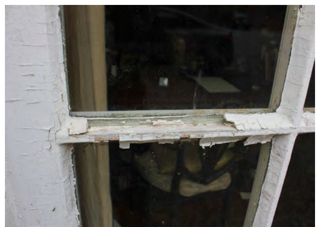
Figure II-165. Missing glazing putty at French doors. (HA, 2015)
