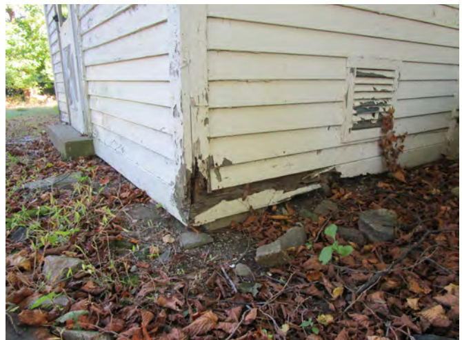
Figure IV-29. Rotted and loose clapboard siding. (HA, 2015)
