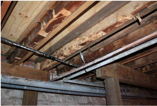
Figure II-321. Termite damaged floor joists under the dining room. (HA, 2015)
