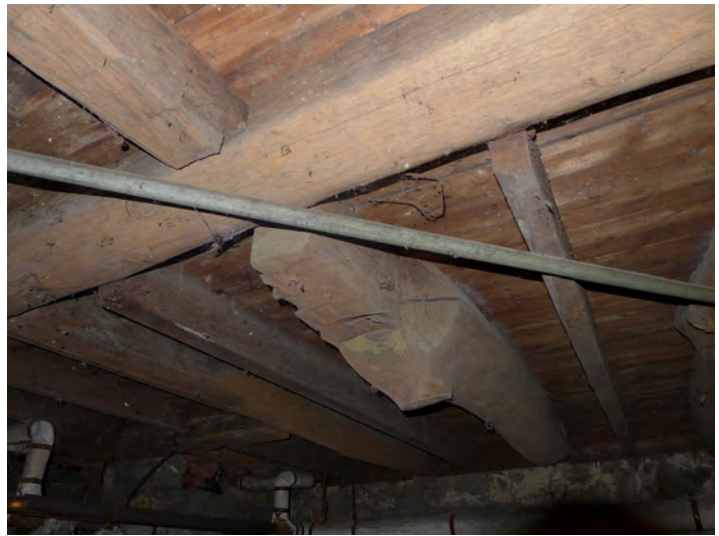
Figure IV-82. Early heavy timbers in 19th century section of the house showing how they were only moderately hewed. (HA, 2015)
