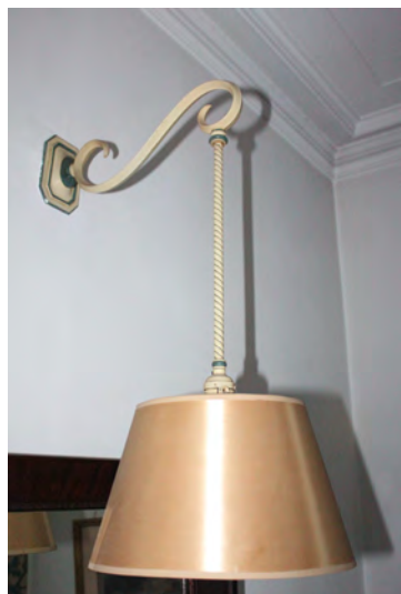
Figure II-310. Light fixture type L19; Wall-mounted bracket with painted finish and hanging single-lamp and shade. (HA, 2015)
