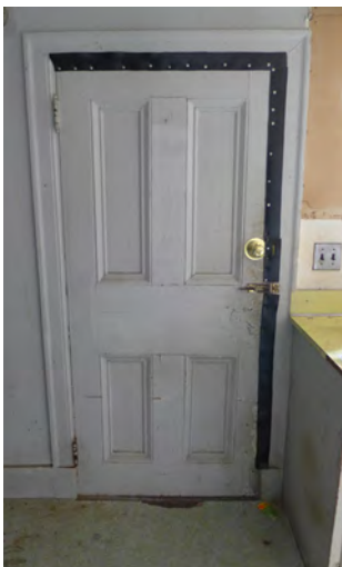
Figure IV-54. Four-paneled door with wide sticking profiles. (HA, 2015)
