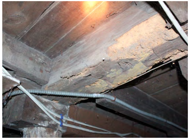
Figure IV-80. Another image showing the heavy timbers and termite damage. (HA, 2015)
