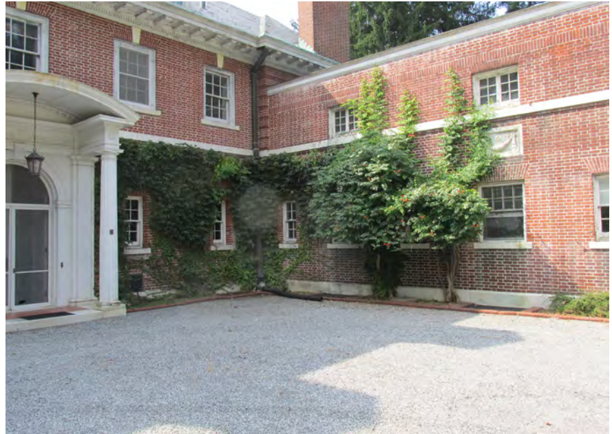
Figure II-137. Extensive vines at intersection of main house and servant's wing. (HA, 2015)
