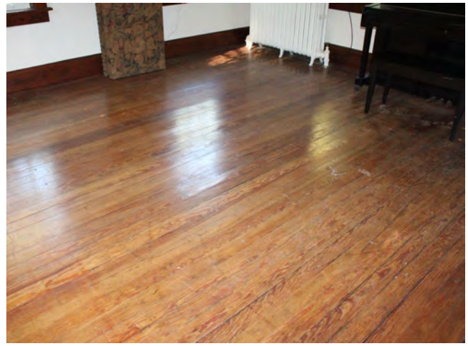
Figure III-59. Resinous finished wood strip flooring. (HA, 2015)
