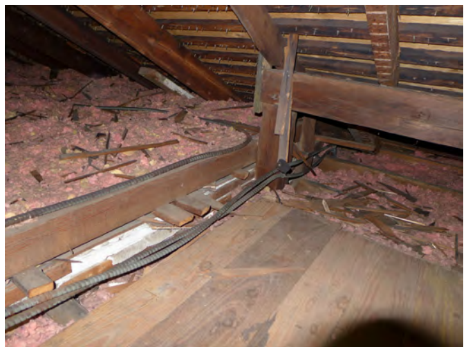
Figure IV-84. The knee wall ends just east of the large cross gable marking a change in construction between the western and eastern portions of the 19th century house. This change in construction suggests that the house likely was added onto several times. (HA, 2015)
