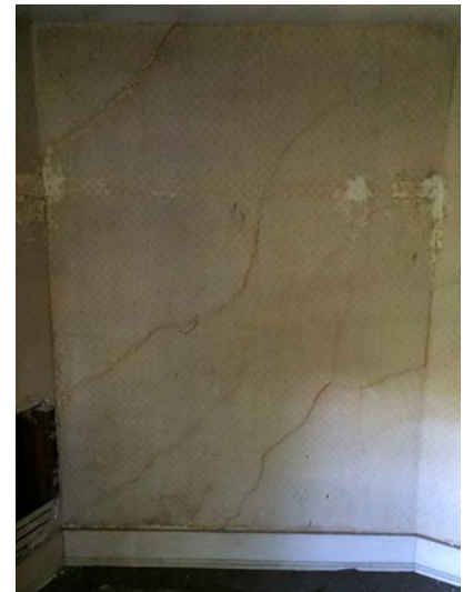
Figure IV-51. Cracks in plaster wall. (HA, 2015)
