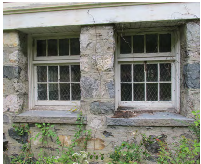
Figure IV-102. Multi-lite windows to the lower level. (HA, 2015)
