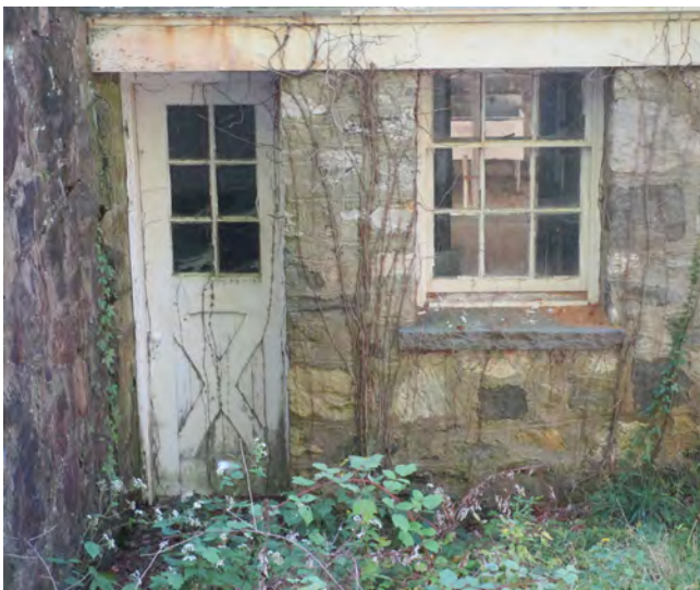
Figure IV-101. Six-lite board and batten door to lower level. (HA, 2015)
