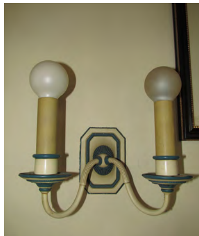
Figure II-308. Light fixture type L17; Painted metal, two-light sconce with glass shade. (HA, 2015)
