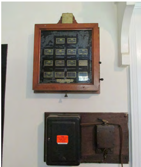
Figure II-315. Original servant's call annunciator box in Pantry (109). (HA, 2015)
