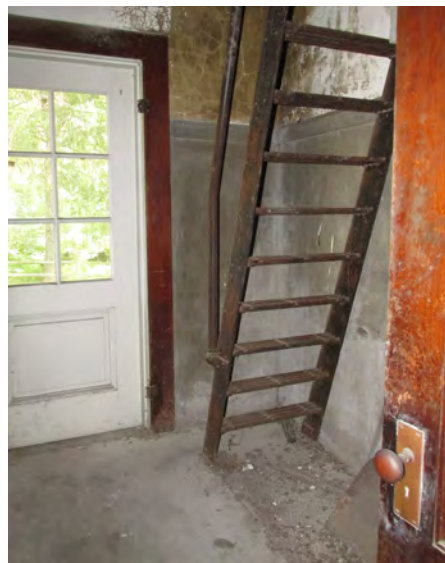
Figure III-92. Ship's ladder in stable wing. (HA, 2015)
