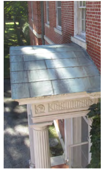
Figure II-154. Flat seam copper roof over east entry. (HA, 2015)
