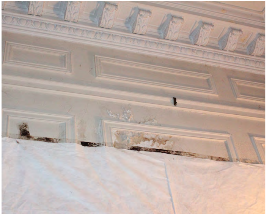
Figure II-224. Water damaged plaster in Dining Room (108). (HA, 2015)
