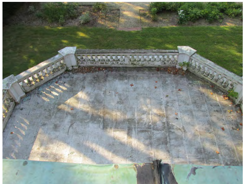
Figure II-151. Flat seam copper roof with asphaltic coating on south porch. (HA, 2015)
