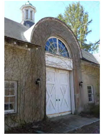
Figure III-50. Flat seam, curved copper roof. (HA, 2015)
