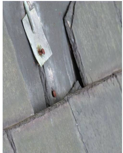
Figure II-149. Corroded ferrous anchors at slate roof. (HA, 2015)
