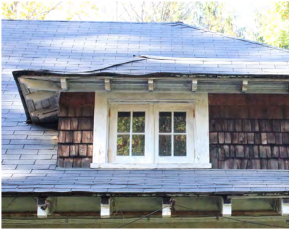
Figure III-48. Asphalt shingle roof. The underlying wood shingles are partly visible at the roof edge and account for some of the waviness. (HA, 2015)
