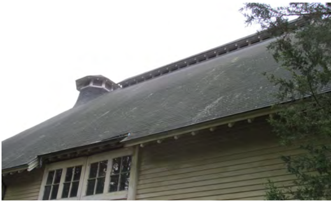
Figure IV-105. Photo of roof showing cupola and ridge vents. (HA, 2015)
