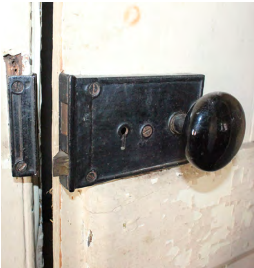
Figure IV-58. Horizontal rim lock, likely from last quarter of the 19th century. (HA, 2015)
