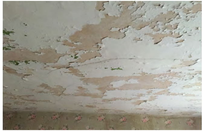
Figure IV-53. Peeling paint in 19th century section of the house. (HA, 2015)
