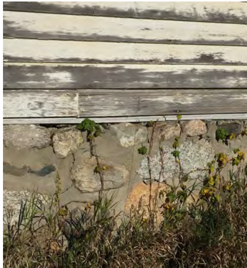
Figure IV-202. Close-up photo of clapboard siding and fieldstone foundation wall. (HA, 2015)
