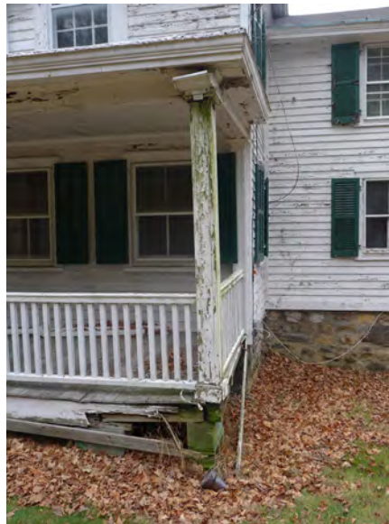
Figure IV-37. Rotted and missing wood at southeast corner of porch. (HA, 2015)
