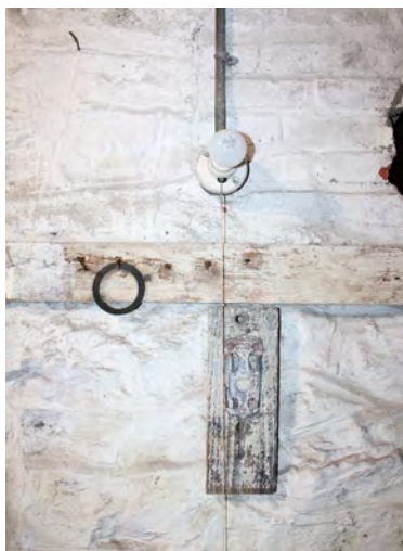
Figure II-292. Light fixture type L1; bare bulb and porcelain socket with pull-chain. (HA, 2015)
