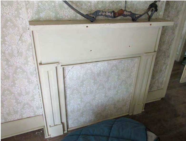
Figure IV-77. Mantel piece in salon/living room in 19th century section of the house. It is not known if the mantel piece is original and no fireplace appears to ever have been constructed based on thickness of the wall and lack of foundation in the basement. (HA, 2015)
