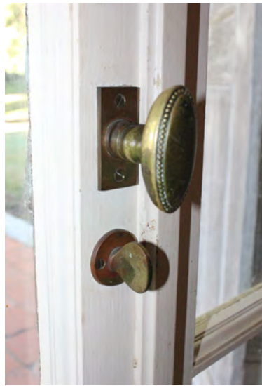
Figure II-184. Bronze knob and turn latch on French doors. (HA, 2015)
