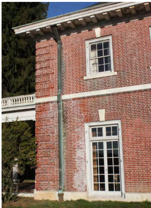
Figure II-133. Efflorescence on west elevation adjacent to downspout. (HA, 2015)
