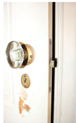
Figure II-281. Lockset with smooth oval glass knob, used in second floor bedrooms. (HA, 2015)
