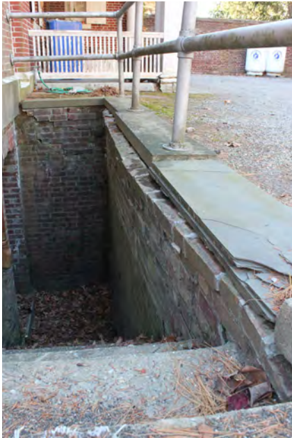
Figure II-136. Displace brick at the basement stair sidewalls. (HA, 2015)
