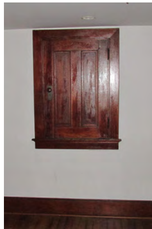
Figure III-71. Two-paneled door. (HA, 2015)
