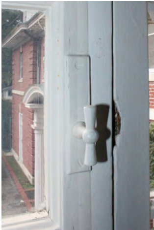
Figure II-189. Casement turn latch. (HA, 2015)
