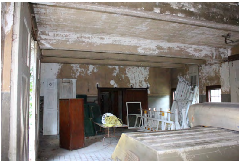
Figure III-63. Cement wainscot and plaster walls and ceilings in carriage room. (HA, 2015)
