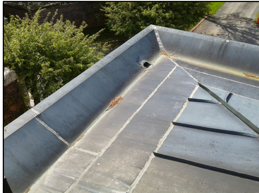
14 PHOTO OF SERVANT'S ROOF SCUPPERS NTS
