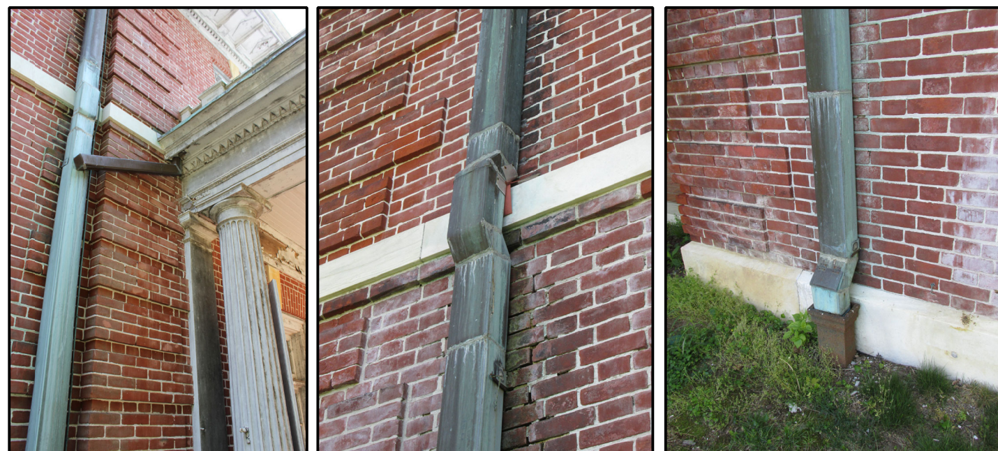
15 PHOTO OF DOWNSPOUT OFFSETS NTS
