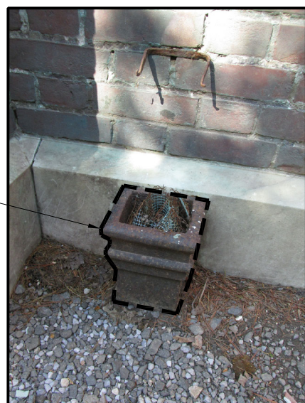
CAST IRON GUTTER RECEIVER
