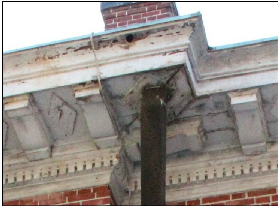
3 PHOTO OF WOOD SOFFIT DAMAGE NTS
