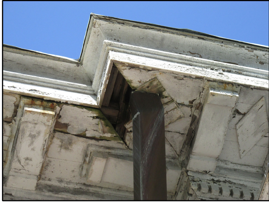
3 PHOTO OF WOOD SOFFIT DAMAGE NTS
