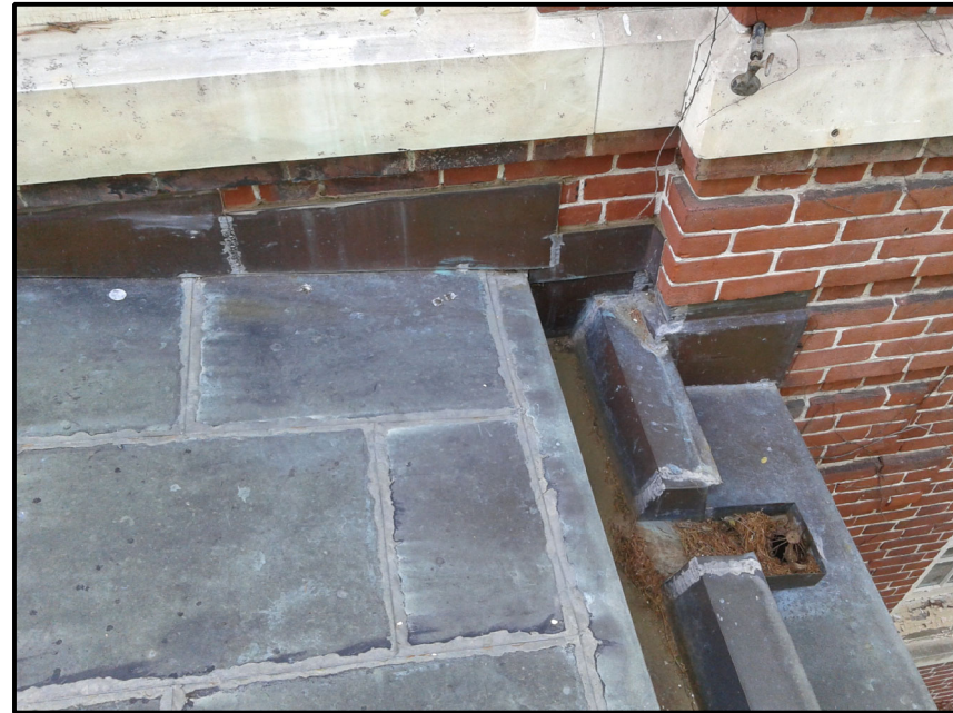
13 PHOTO OF SERVANT'S PORCH GUTTER NTS
