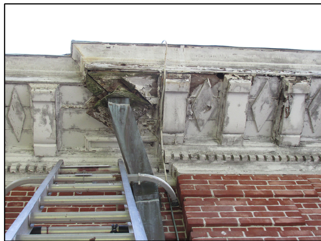
3 PHOTO OF WD SOFFIT DAMAGE SCALE: 1/8"=1'-0"
