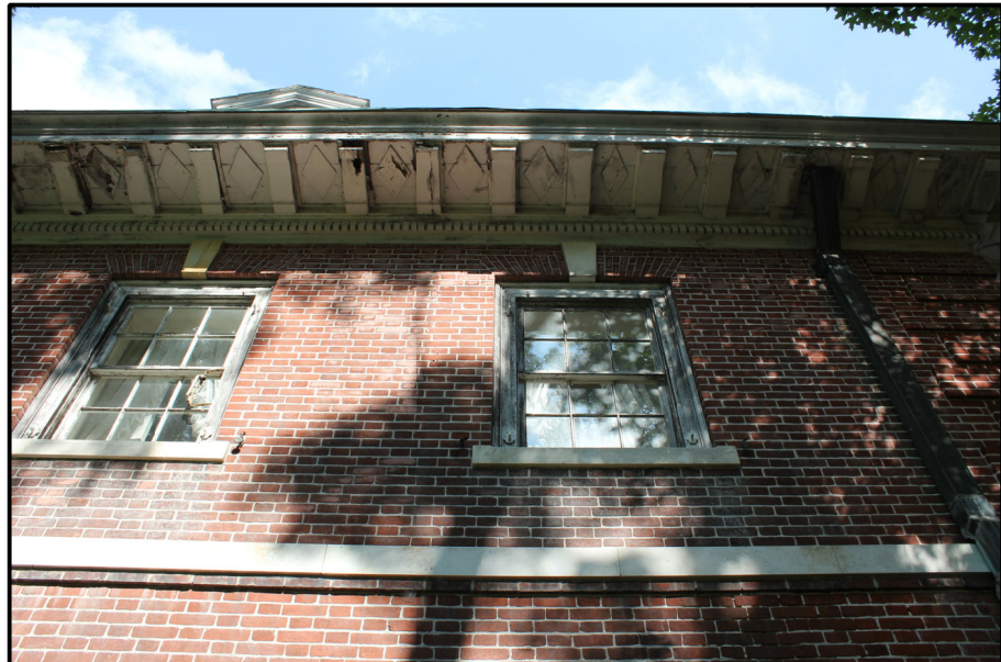
5 PHOTO OF WOOD SOFFIT DAMAGE NTS PHOTOS ARE FOR REFERENCE ONLY.
