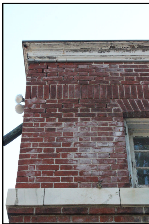
4 SEVERELY ERODED BRICK SCALE: 1/8"=1'-0"
