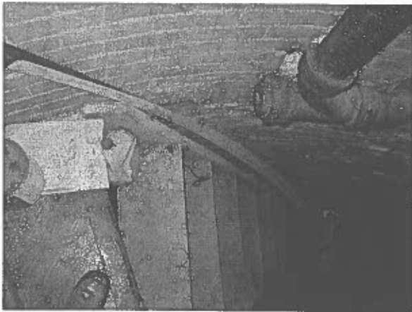
A-3. LIGHTHOUSE CELLAR LANDING SHOWING THE DILAPIDATED WOODEN STAIRCASE.
