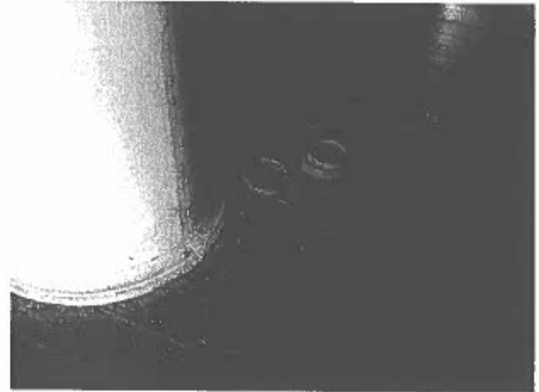
A-16. HOT AND COLD WATER PIPE SLEEVES ON FLOOR LEVELS 1 THROUGH 4.
