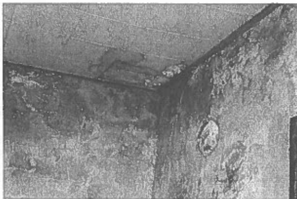
A-10. STAINED AND DILAPIDATED CEILING PANELS IN FORMER OFFICE SPACE.
