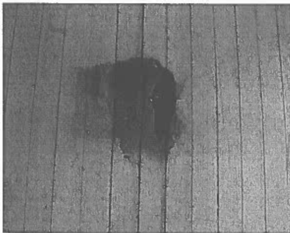
A-9. FIRE DAMAGE ON FOURTH FLOOR WOODEN FINISHED FLOOR.
