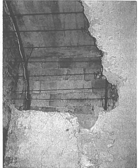
A-2. MISSING CHUNKS OF STUCCO IN VAULTED CEILING EXPOSING RUSTED "C" CHANNELS.
