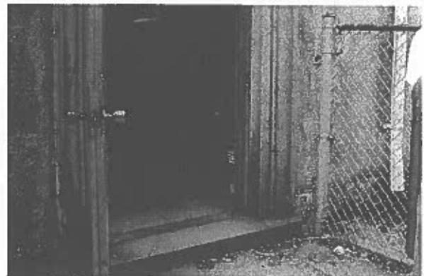
A-13. BIOLOGICAL GROWTH AND STRUCTURAL CRACKS ON EXTERIOR MASONRY WALLS.
