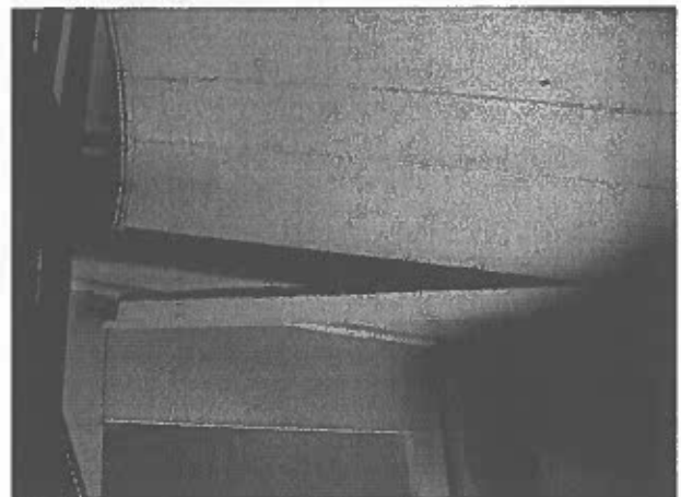
A-10. FALLING WOODEN PLANK CEILING PANELS.
