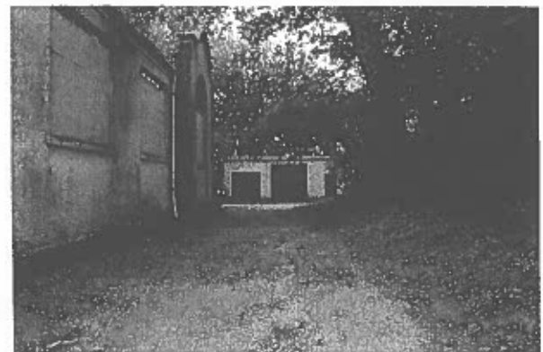
A-11. BOARDED UP WINDOWS AND BIOLOGICAL GROWTH ON EXTERIOR MASONRY WALLS.
