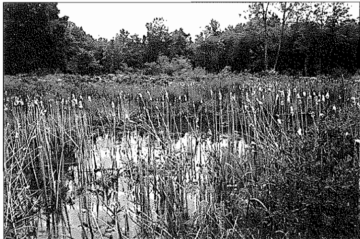
"Wet" detention basins and artificial wetlands, such as these at the Westchester County Airport, control flooding and improve the quality of stormwater runoff.
